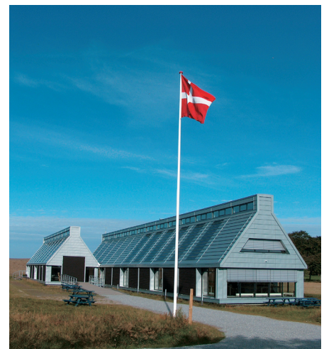
The walls and windows of the Energy Academy are highly insulated to minimize energy consumption and the building is heated by the local straw-fired district heating plant. Photo: Samsø Energy Academy
