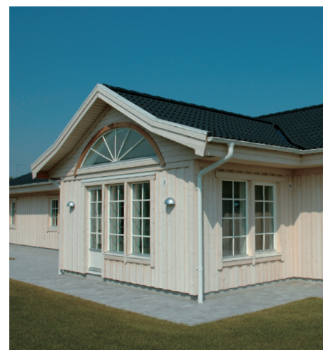
THE ECO-FRIENDLY HOUSES AT HERFØLGE LOOK LIKE ORDINARY ONES, BUT USE APPROXIMATELY 50% LESS ENERGY.
