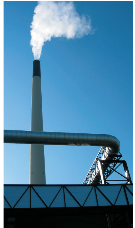
The flue gas treatment is so efficient that Vestforbrænding operates far below the environmental limit values.
